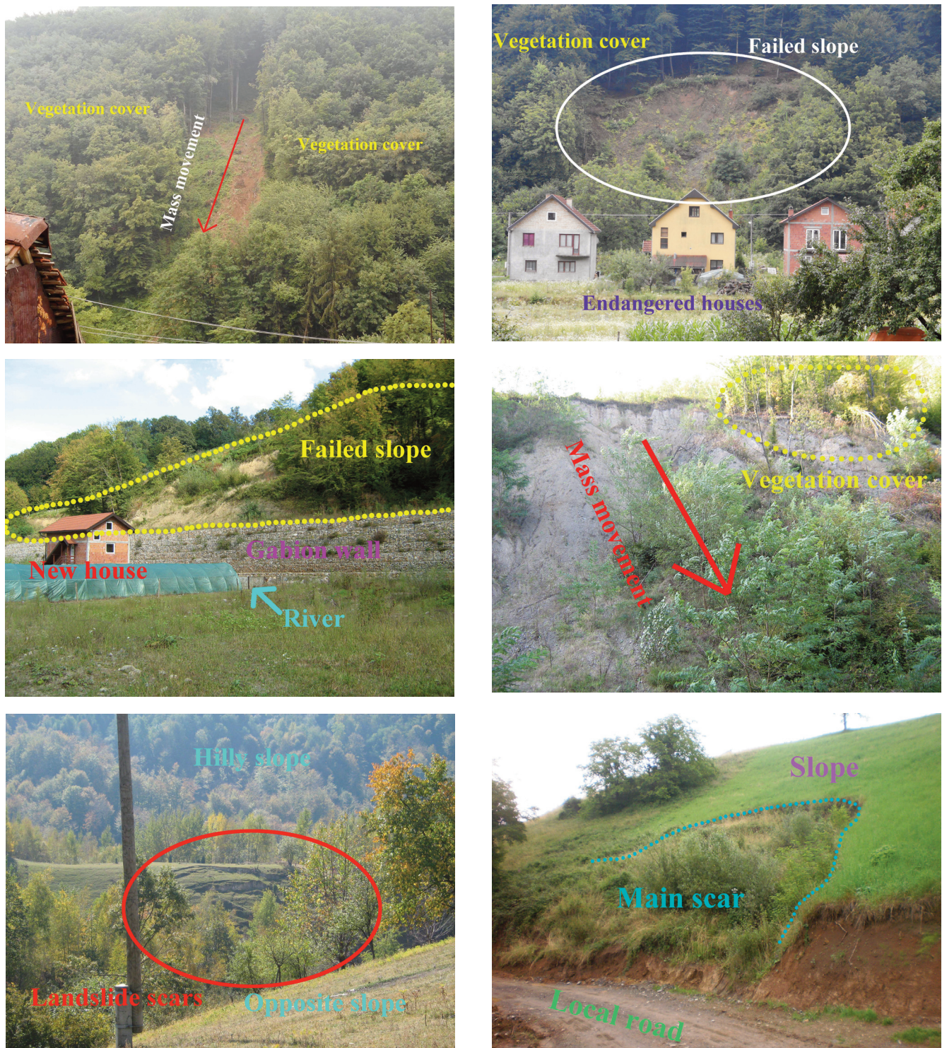
Fig. 3. Landslides in Krupanj area.
